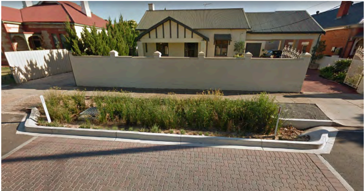
Figure 5.8—Bioretention System (Raingarden), Tarragon Street, Mile End
